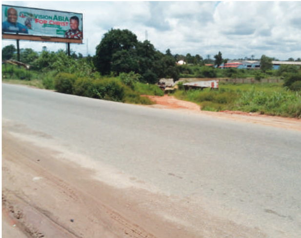
Completed Mbaise+Ngwa road at Imo River
